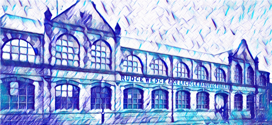
Located at Pelham Works, a historical building built in the 1890s for Rudge Wedge Cycles.
